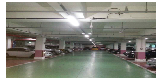
Fluorescent lights after LED dimmer installation
