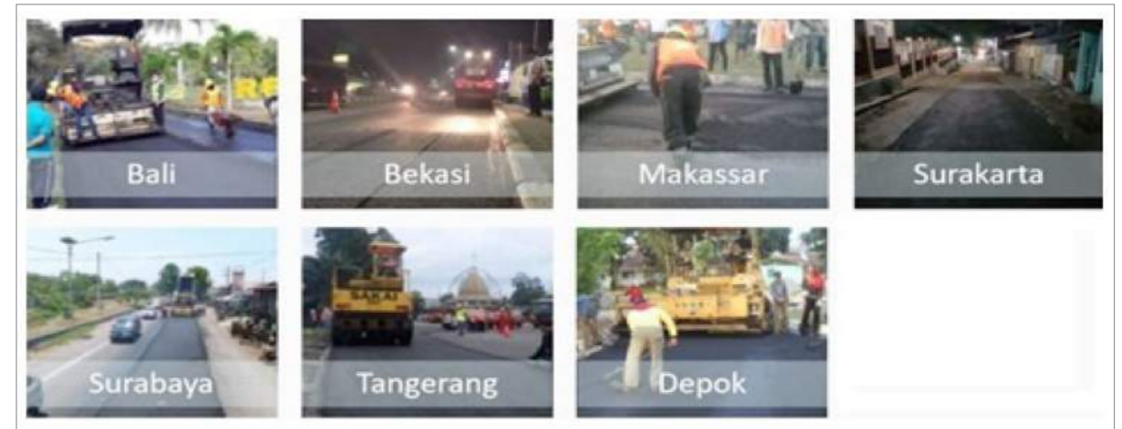
Figure 25 Indonesia's Asphalt Plastic Implementation in 7 cities in Indonesia
